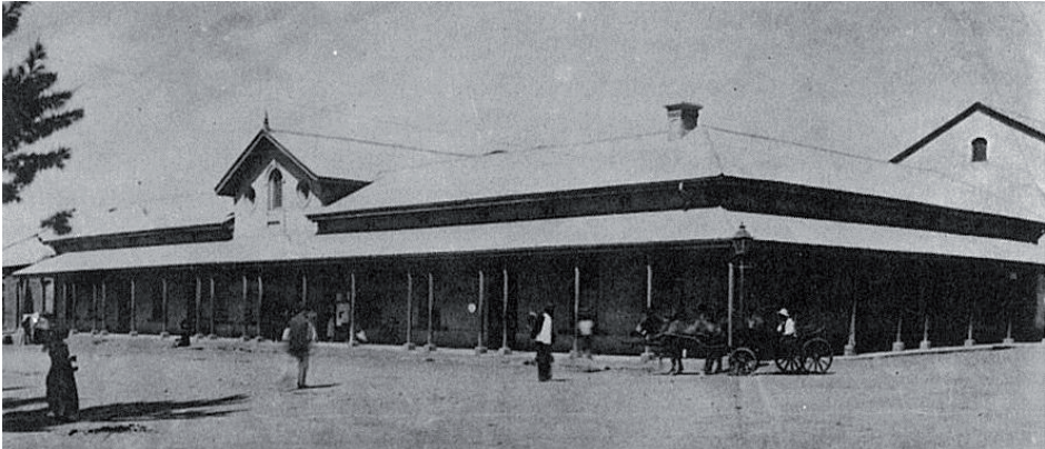
Image 3: Graaff-Reinet Magistrates Court (incorporating Post Office)
