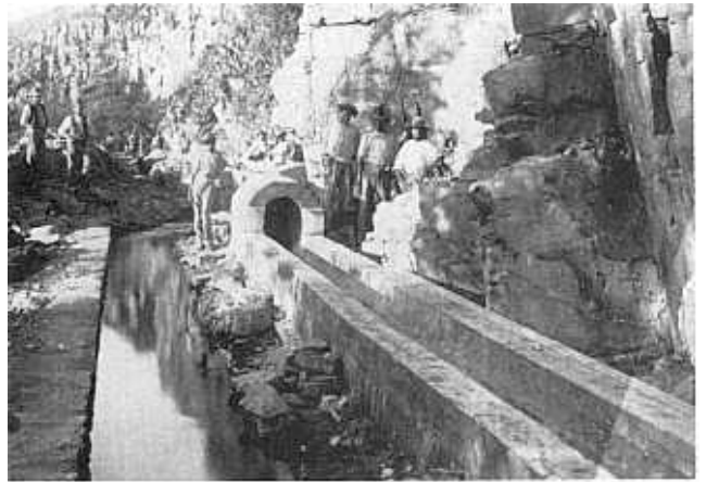
Construction of the Mackie's Pit culvert, 1883-1884.
