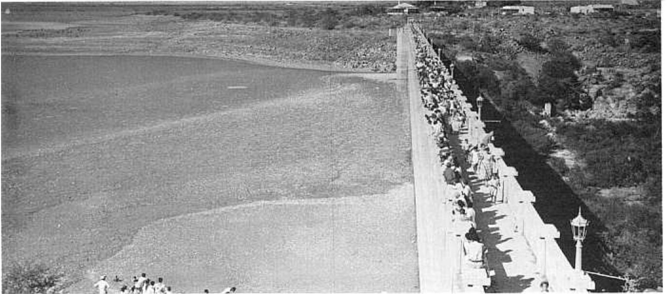
The Van Ryneveld's Pass Dam empty for the first time, 1957.
