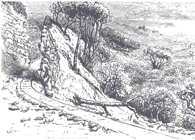
A short railway embankment, Ross's Camp.
