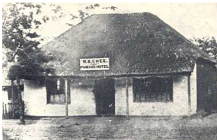
Phoenix Hotel, Durban, ca. 1860, showing early wattle and daub construction with thatched roof.
